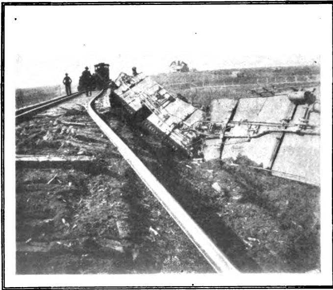
WRECK ON THE FRISCO, FEBRUARY 10, 1907, NEAR DAVIDSON, OKLA.—VIEW FROM REAR, LOOKING TOWARD ENGINE
