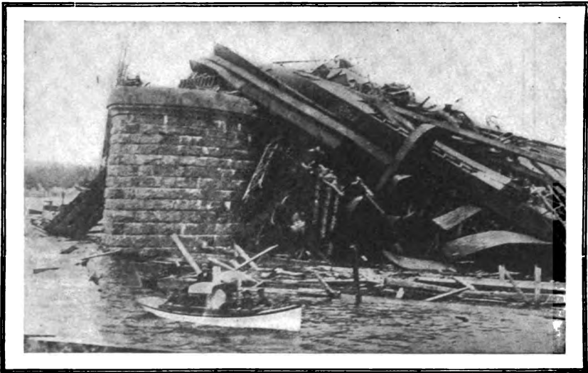
THE QUEBEC BRIDGE DISASTER
