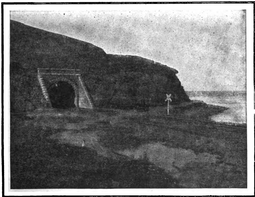
ENTRANCE TO TUNNEL NO. 4, THE LONGEST—BAY SHORE CUT-OFF
