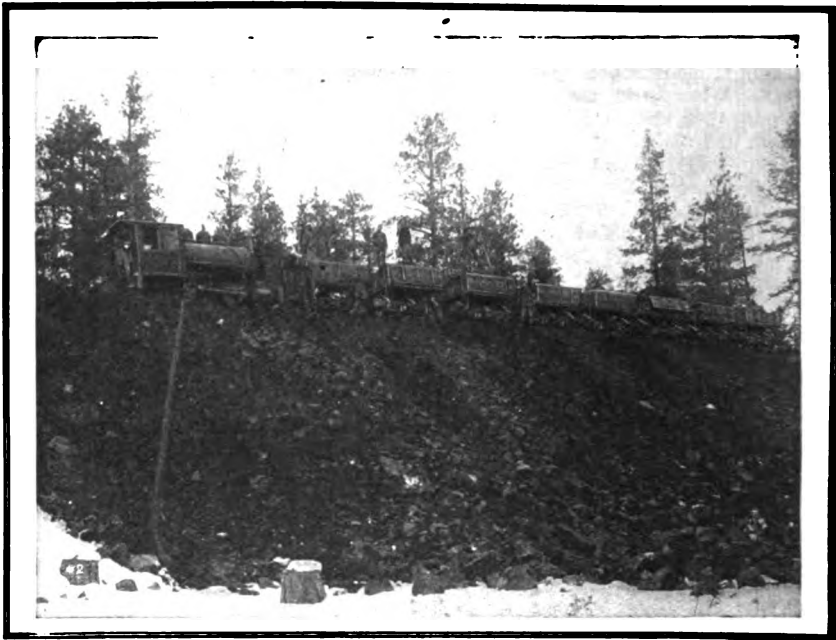
HEAVY FILL BEING MADE FROM THE "SUMMIT CUT"—CALIFORNIA & NORTHEASTERN RAILROAD
